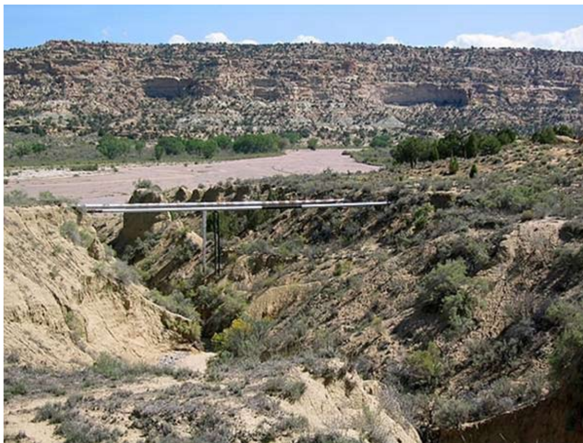
Figure 4. This New Mexico pipeline crosses the channel near the elevation of the highest terrace, which places it above even the most extreme flood events.
