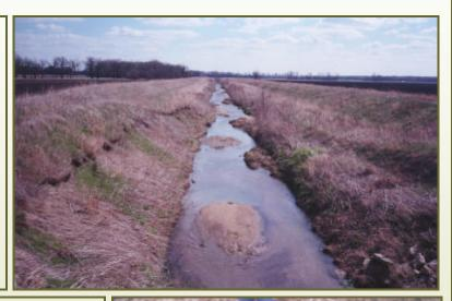
A sheadcuts move upstream, the deepening channel remains narrow with high water velocities. Eroded material is transported downstream where water velocity slows due to a wider or meandering channel with a flatter slope. When water velocities are reduced, excess sediment is deposited, constricting the channel and increasing flood problems.
