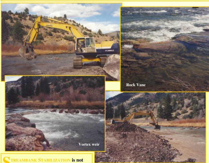
rebuilding a stream channel, but only slowing or stopping the erosion along a stream bank.
