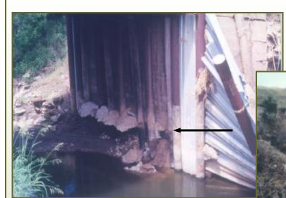
Channel incision is often evident at bridges or other structures constructed in stream channels.
