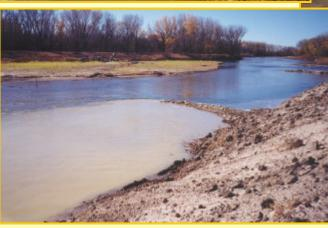
Reduced water velocities on the downstream side of bendway weirs result in sediment deposition near the bank.
