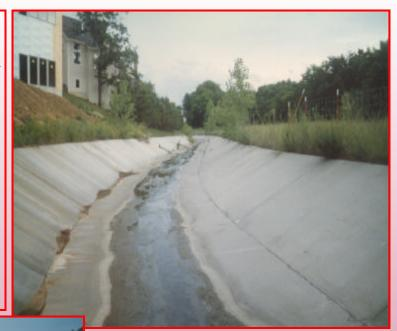
Constructed stream channels are often designed for flows greater than bankfull. Normally, this type of channel is too wide to efficiently move sediment during flows at bankfull or less. These channels usually require high construction and maintenance cost.
