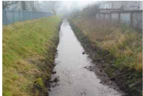
Mayes Brook : An example of a proposed project with associated full information sheet 1
