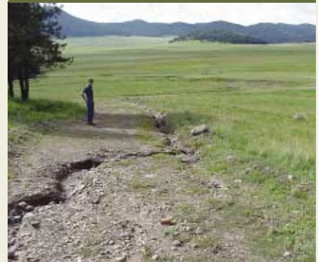
Figure 50. Without maintenance and proper management, roads will continue to degrade and supply sediment to adjacent riparian areas.
