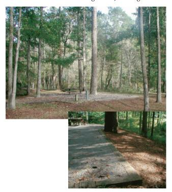
Figure 67–Site cover material is 1/4 inch and less crushed limestone for accessibility. Each campsite area is framed in timber.
