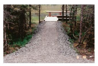
Figure 63–This trail allows water to flow through it, preserving the wetland and providing a dry walking surface.
