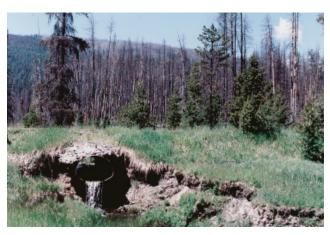
Figure 57–Drainage patterns changed when a road was built across this meadow. The water can drain through only a few culverts, which concentrates the outflow and causes down cutting that has lead to an incised stream.
