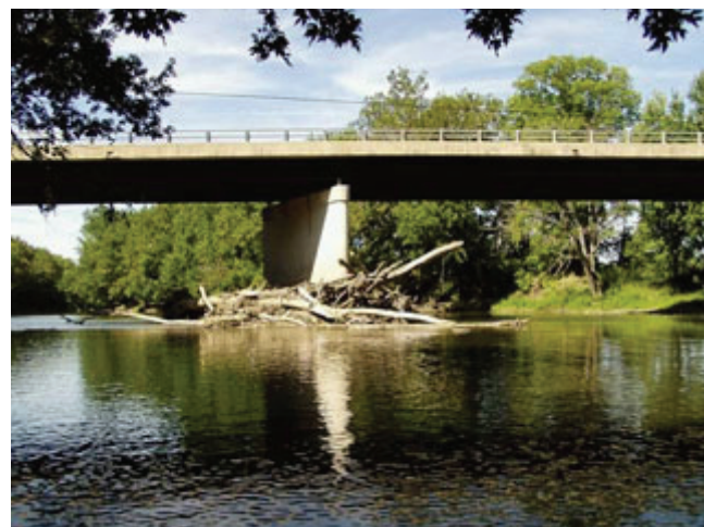
Figure TS14J-2 White River, IN, with large woody debris ( Photo courtesy of USGS )
